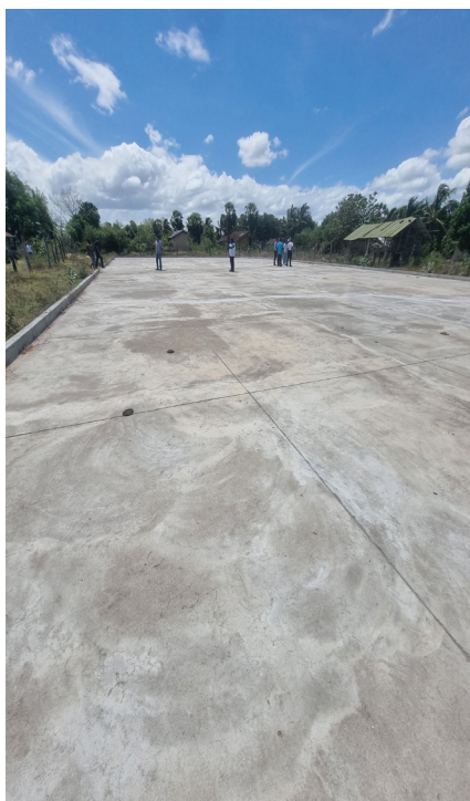
Constructed 10,000 sqft Paddy Drying Bed
